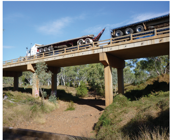
Bridge across the Cloncurry River Anabranh, mid 2012
