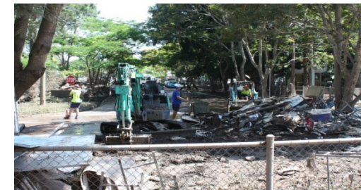
Recovery occurring across one of the many affected Qld schools
