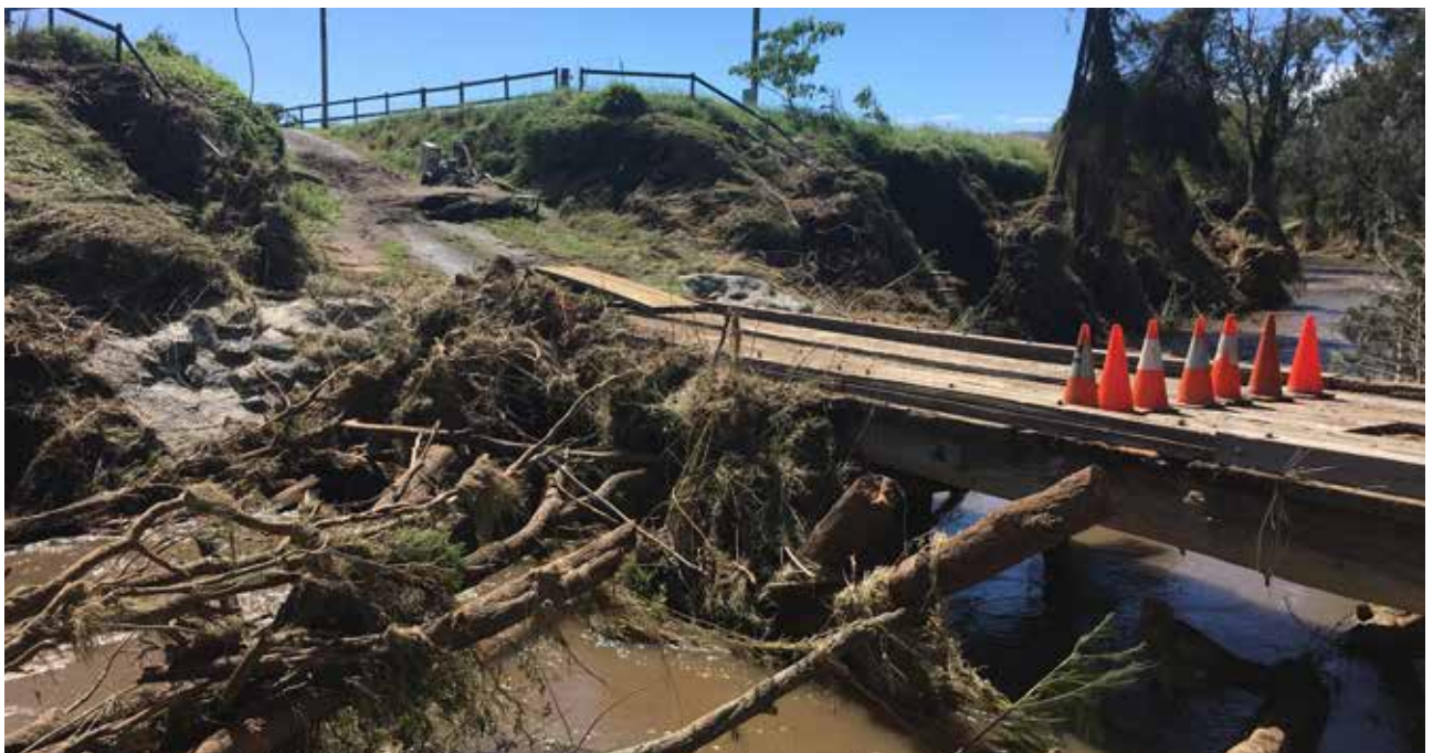
Haack Road Bridge in the Scenic Rim was damaged by high velocity floodwaters in Christmas Creek
