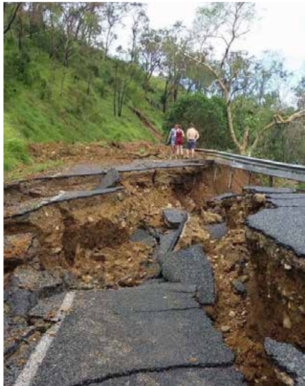
Damage to Marlborough – Sarina Road, Sarina
