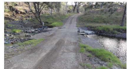
Photo demonstrates overview and asset scouring
