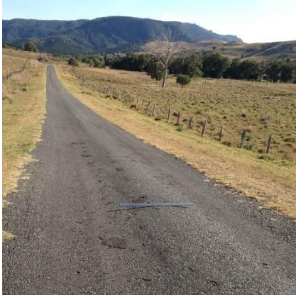
Use a straight edge to demonstrate the nature and extent of damage to the asset
