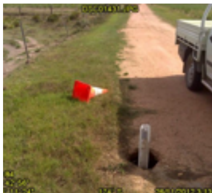
Use a measure, ruler or other available prop to demonstrate extent and nature of damage and support proposed scope of works – e.g. sinkholes/blowholes
