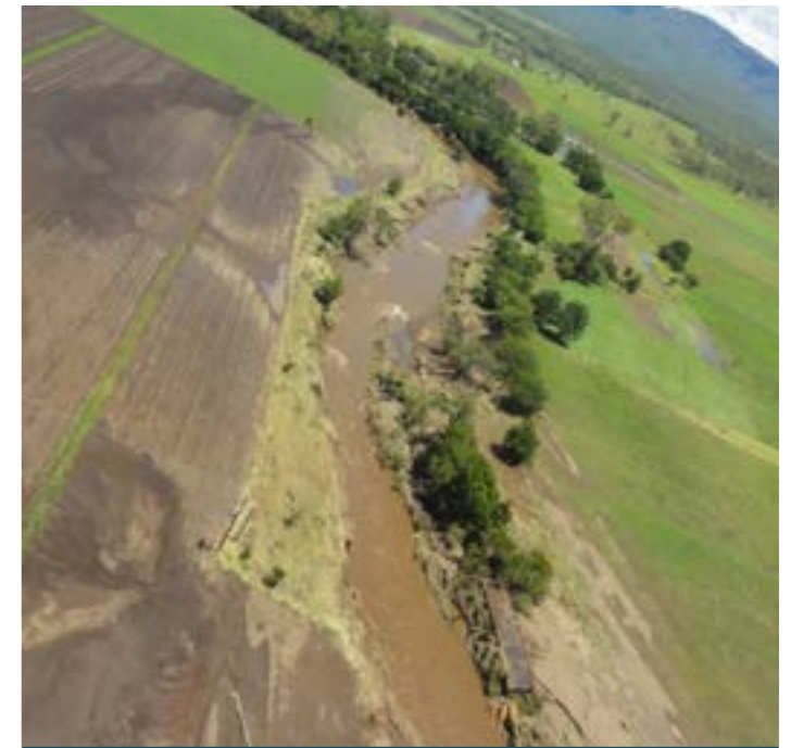
Lockyer Valley, Thornton School Bridge – 2013 flood
