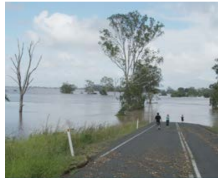
Somerset, Lowood – 2011 flood
