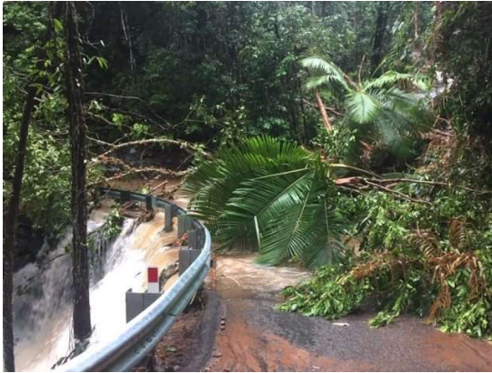
Damage to Alexandra Range, Cape Tribulation Road
