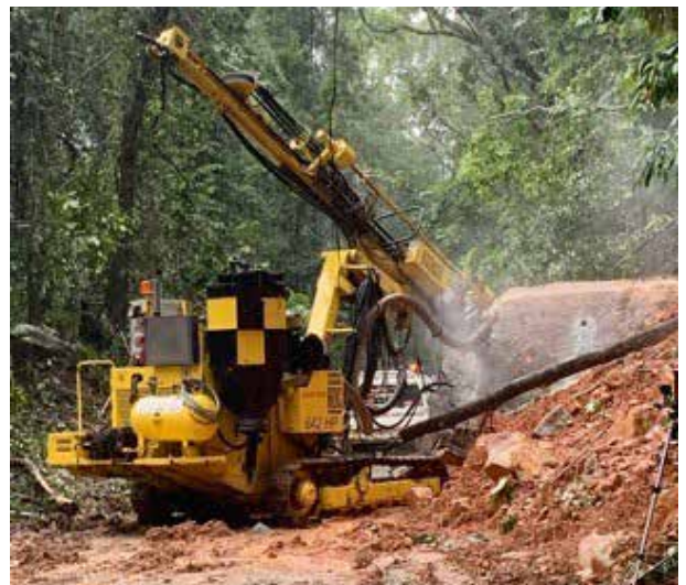
Emergency works to break down boulders - Mount Spec Road
