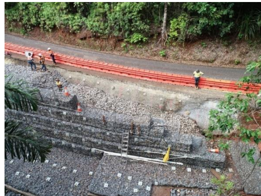
Once strengthening works have been finished, restoration of the missing road lane could be completed. The Douglas Shire Council, consultants and contractors worked hard to repair the road, however the poor soil conditions have hampered progress and significantly increased the scope of work beyond what was initially expected
