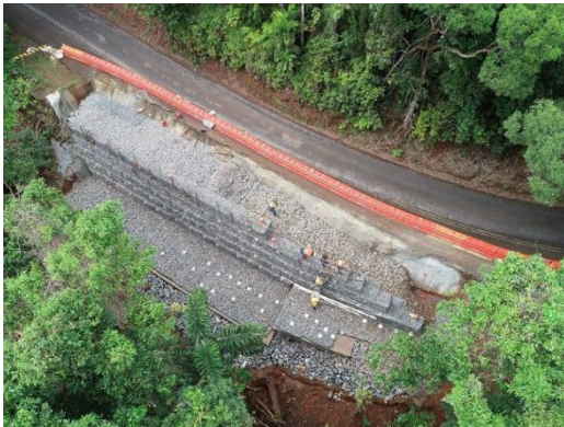
Contractors have been drilling specialised soil nails and spraying it with concrete to keep the area secure
