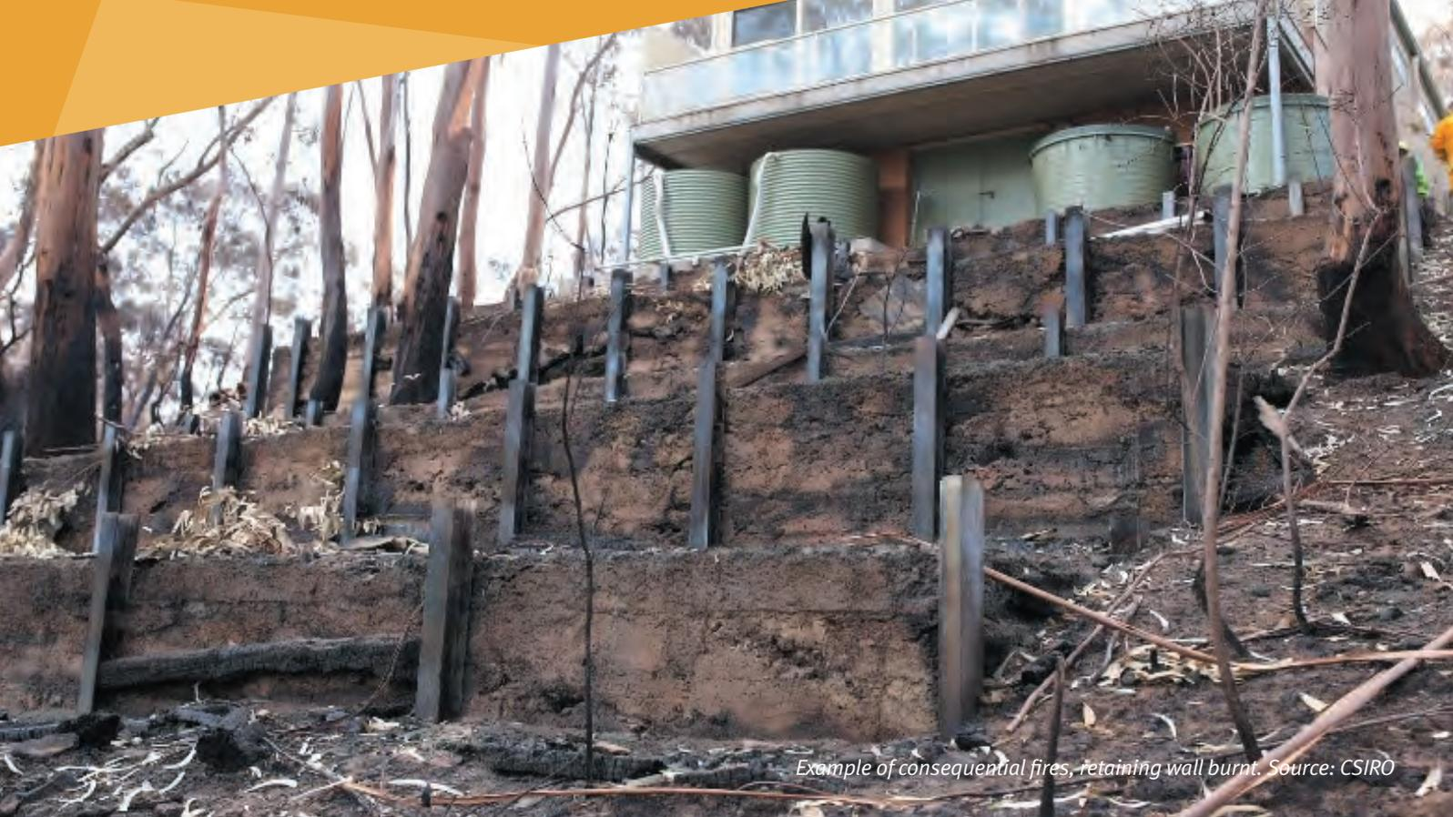
*Example of consequential fires, retaining wall burnt. Source: CSIRO*
