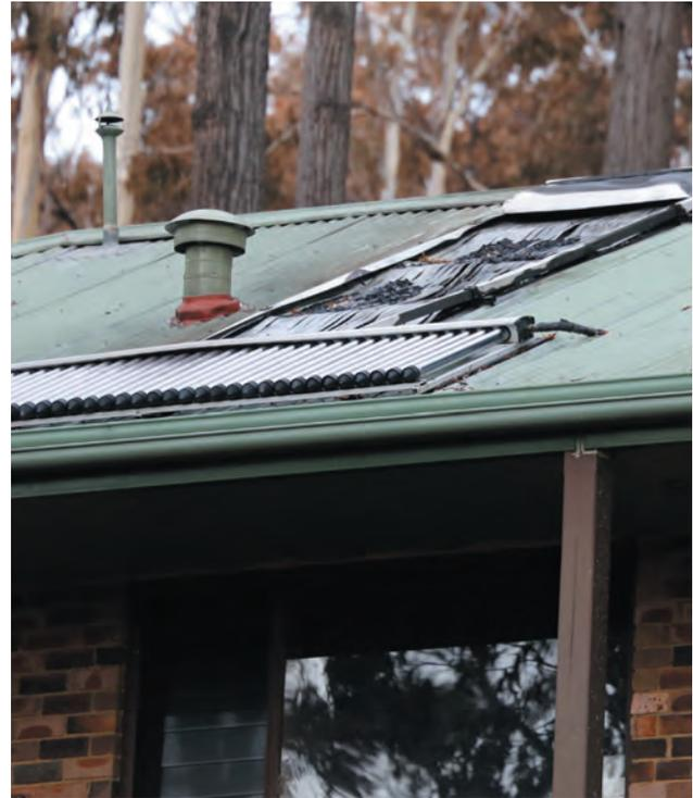
*Example of roof perforation and combustible elements on roof.*
