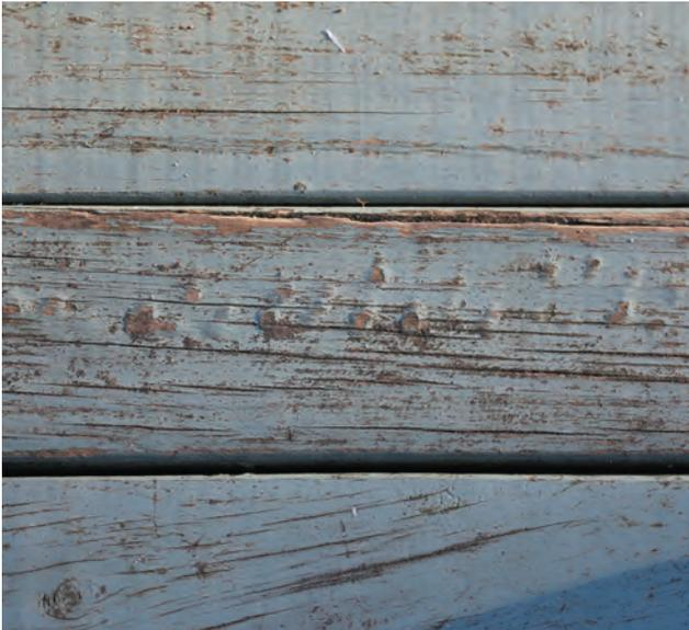
*Damaged deck is vulnerable to ember attack.
