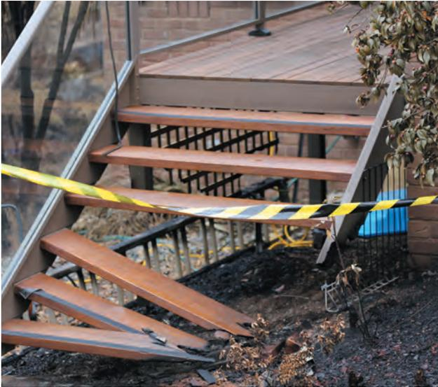
*Potential issue with exit path on fire damaged stairs.
