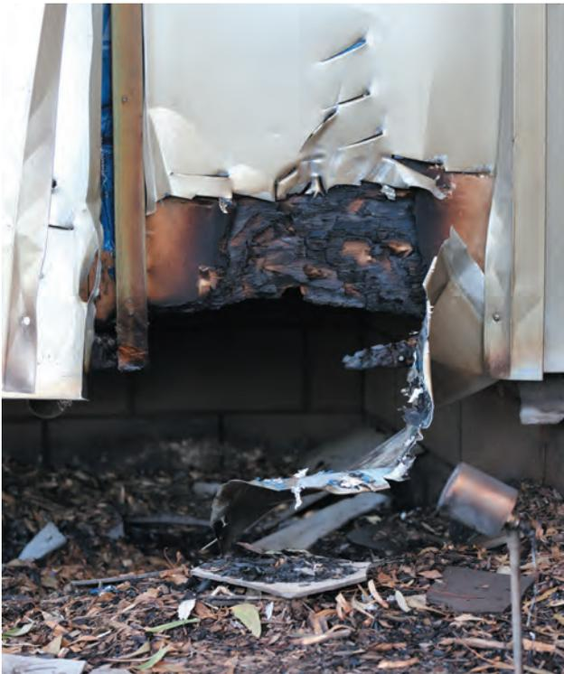
Damaged wall from burning vegetation. Source: CSIRO
