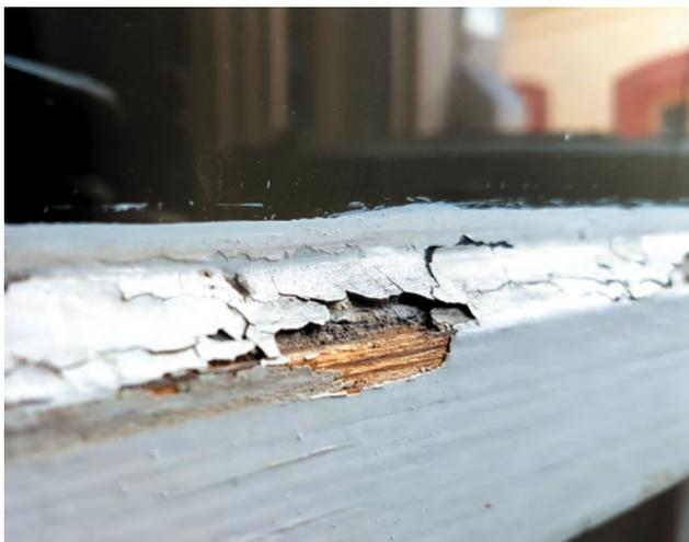
*Damaged or decaying timber frames are vulnerable to ember attack.*
