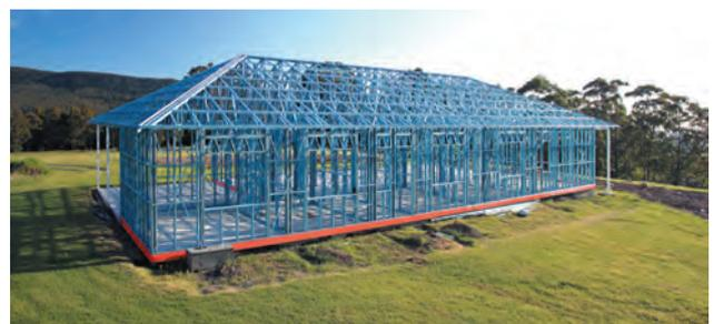
Example of house built using non-combustible framing material (steel frame). Source: KNK Builders
