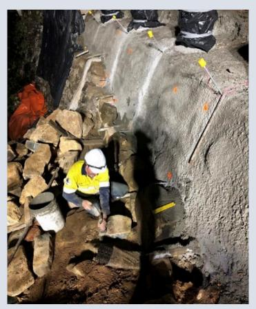
Image: Mount Spec Road – stonemason working on the heritage-listed drystone wall.
