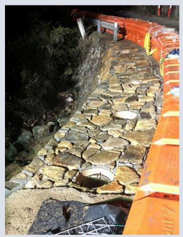
Image: Mount Spec Road - restored drystone wall.
