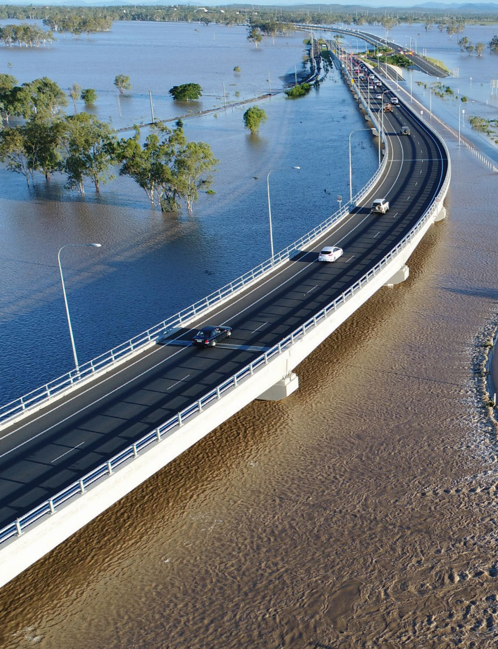
Yeppen Floodplain Crossing, Bruce Highway following Ex-Tropical Cyclone Debbie.
