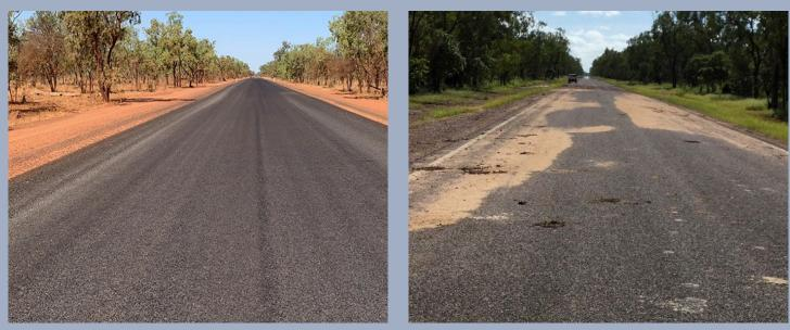
Images: Burke Developmental Road (left): completed betterment works. (Right): silt on road following Tropical Cyclone Imagen.
