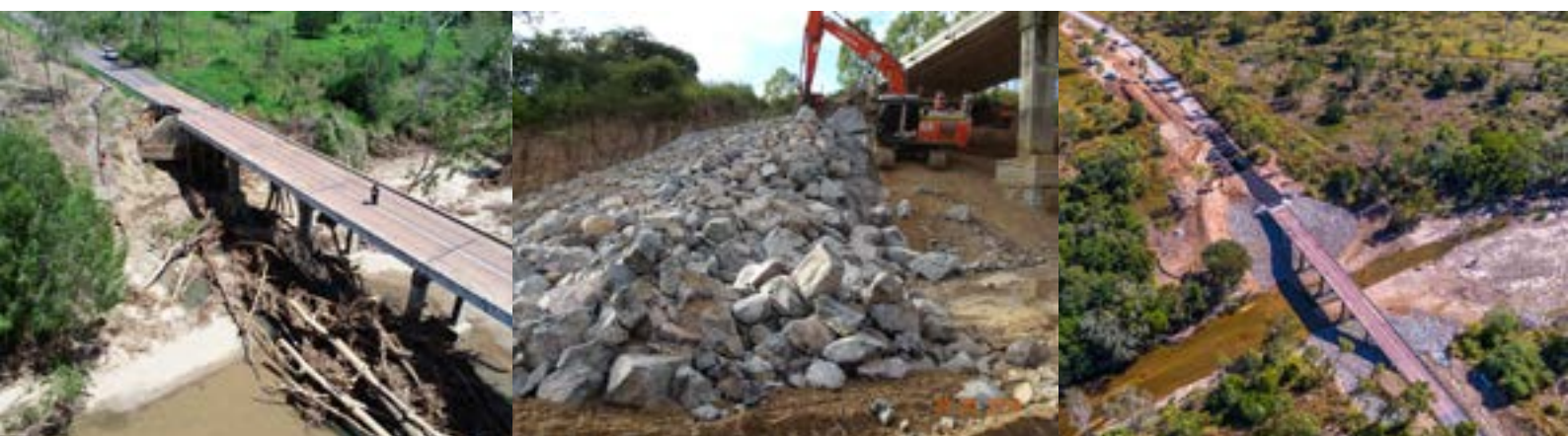
Image (l-r): Damage to Alice River Bridge N&FN Monsoon Trough, reconstruction process, ariel view completed works.
