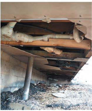
Underfloor damage caused by burning garden bed, supressed by fire agency before it burnt into the house. Source: CSIRO
