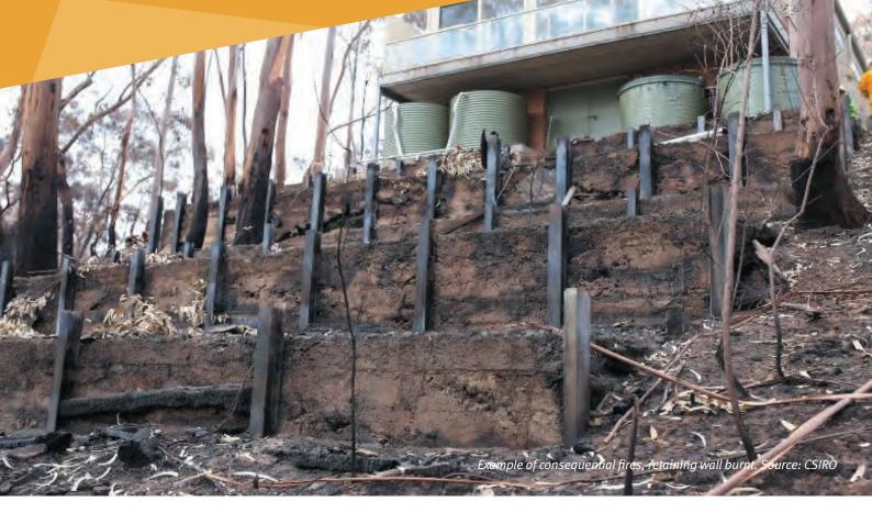
House loss because of bushfire is a complex phenomenon that involves several mechanisms related to the ignition and propagation of fire. When bushfires spread into an urban (or built-up) area, bushfires will impact both houses and their surrounding elements (e.g. fences, retaining wall, cars and sheds). Some of these surrounding elements will ignite and present additional impacts to buildings beyond the bushfire itself. This burning of surrounding elements is called a **consequential fire**.
