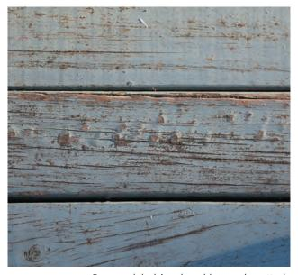
Damaged deck is vulnerable to ember attack. Source: CSIRO
