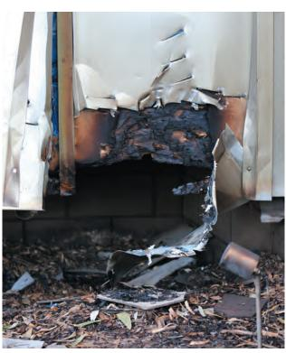
Damaged wall from burning vegetation. Source: CSIRO
