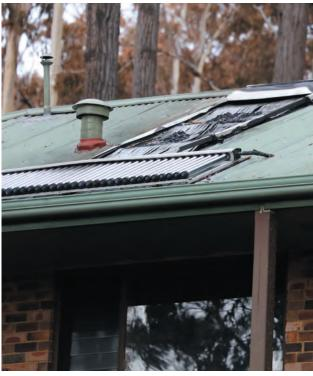
Example of roof perforation and combustible elements on roof.
