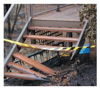
Potential issue with exit path on fire damaged stairs. Source: CSIRO
