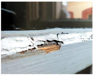
Damaged or decaying timber frames are vulnerable to ember attack.
