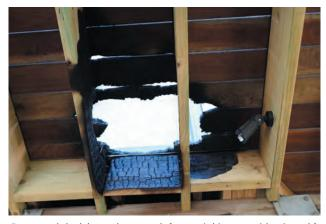
Damaged deck by ember attack (potential issues withexit path).
