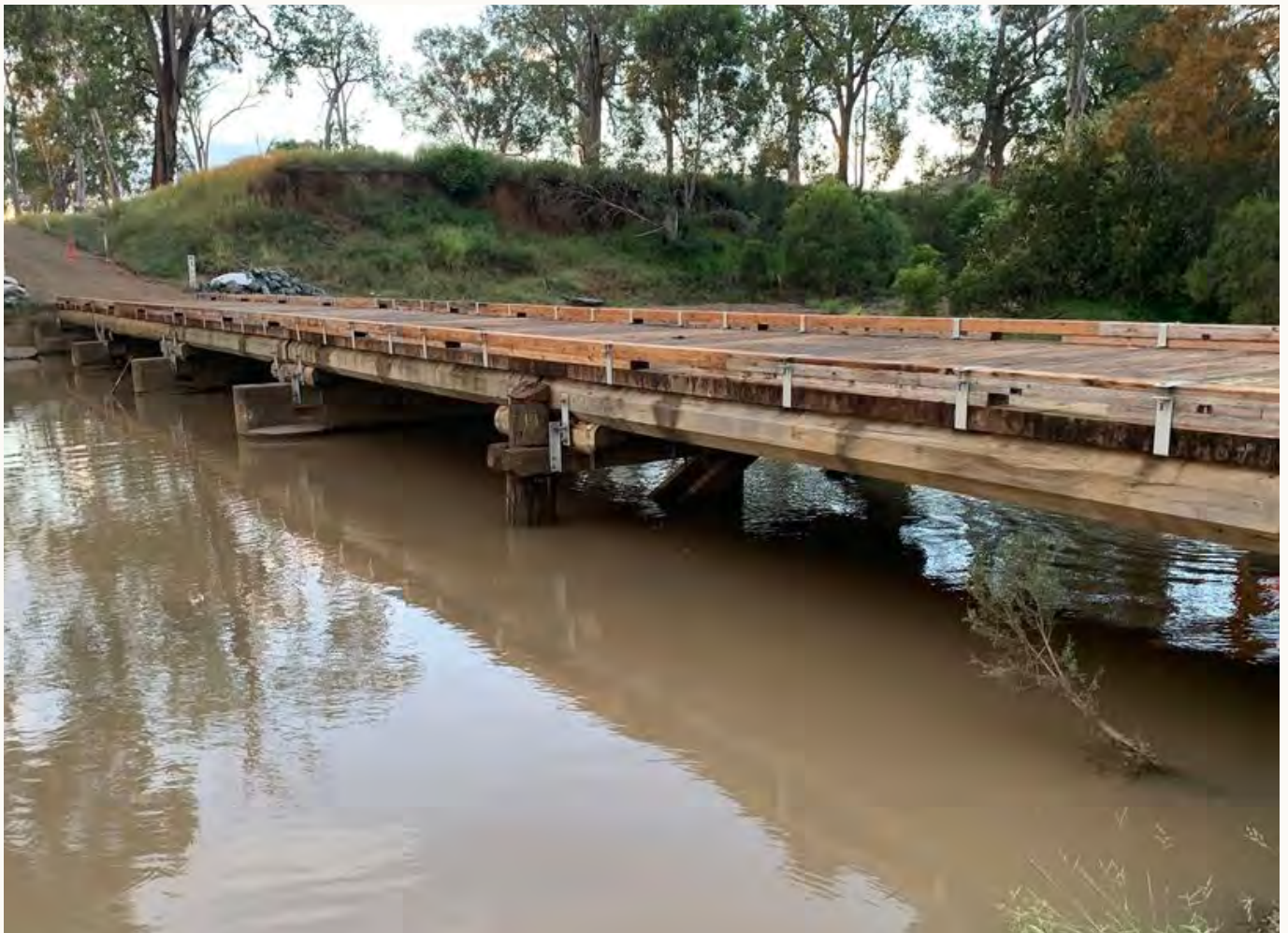
Image: Mountain Creek Bridge, North Burnett.
