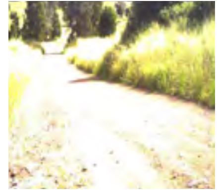
Unable to see damage
