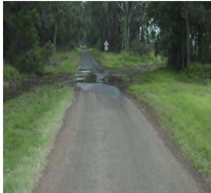
No event damage visible
