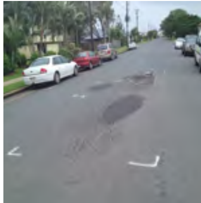
Use spray mark ups to show event damage and proposed scope of works
