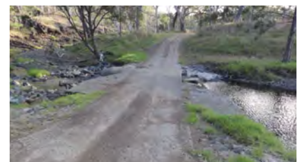
Photo demonstrates overview and asset scouring
