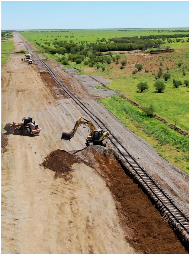
Image: Repair works to Mount Isa rail line following damage during the 2019 North & Far North Queensland Monsoon Trough.
