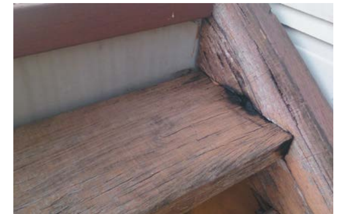
Ember attack in re-entrant corners. Source: CSIRO
