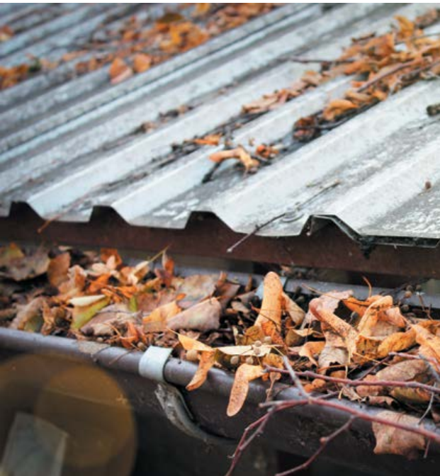
Debris accumulation in gutter.
