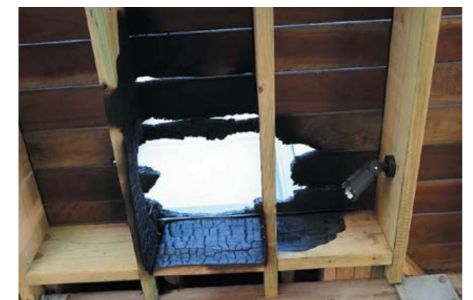
Damaged deck by ember attack (potential issues with exit path). Source: CSIRO
