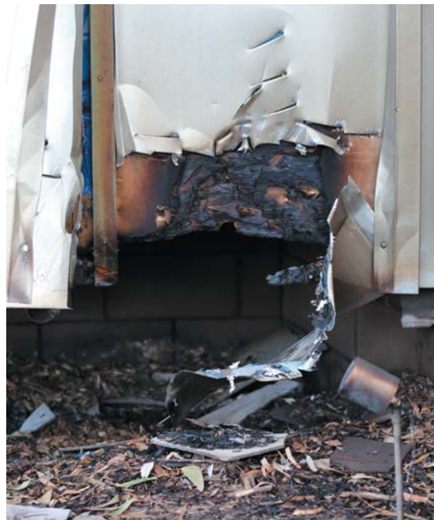
Damaged wall from burning vegetation. Source: CSIRO
