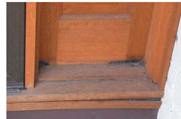
Embers attack in re-entrant corners. Source: CSIRO
