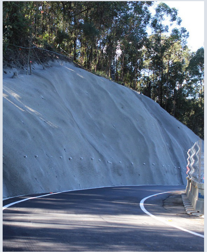
Beechmont Road – stabilisation works (July 2022)
