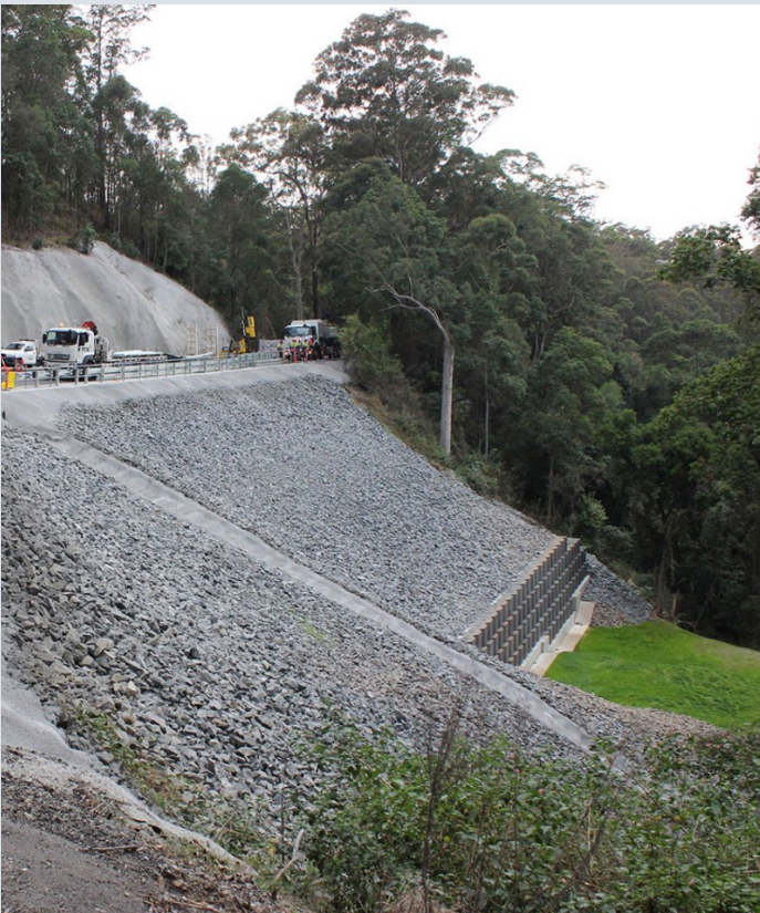
Beechmont Road – completed downslope stabilisation works (August 2023)
