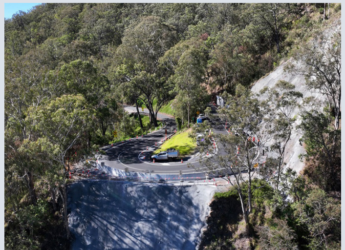
Lamington National Park Road – completed stabilisation works (May 2023)
