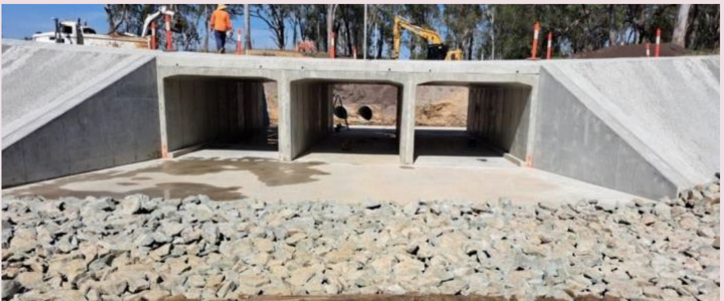
Completed works (November 2024)
