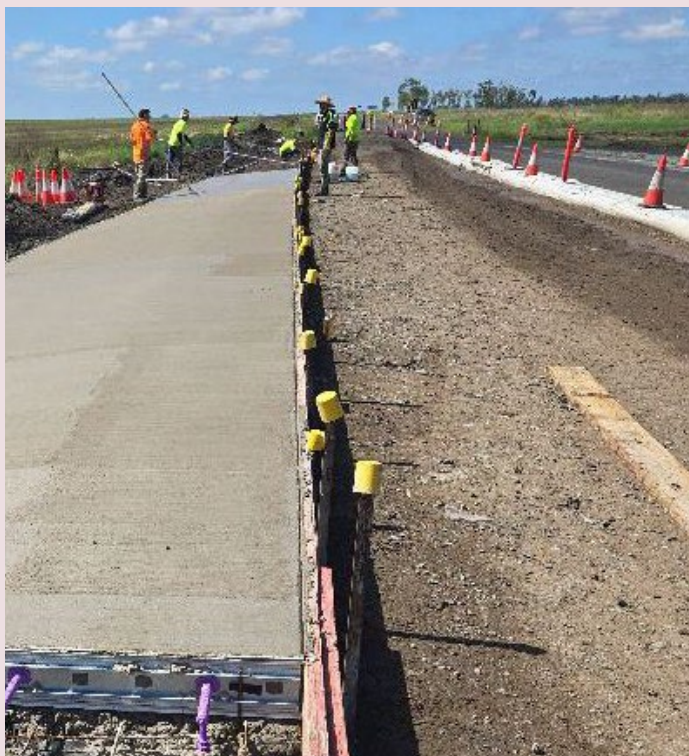
Betterment works in progress at Ashall Creek (December 2024)
