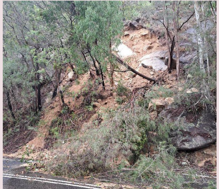
Landslip following TC Jasper (December 2023)
