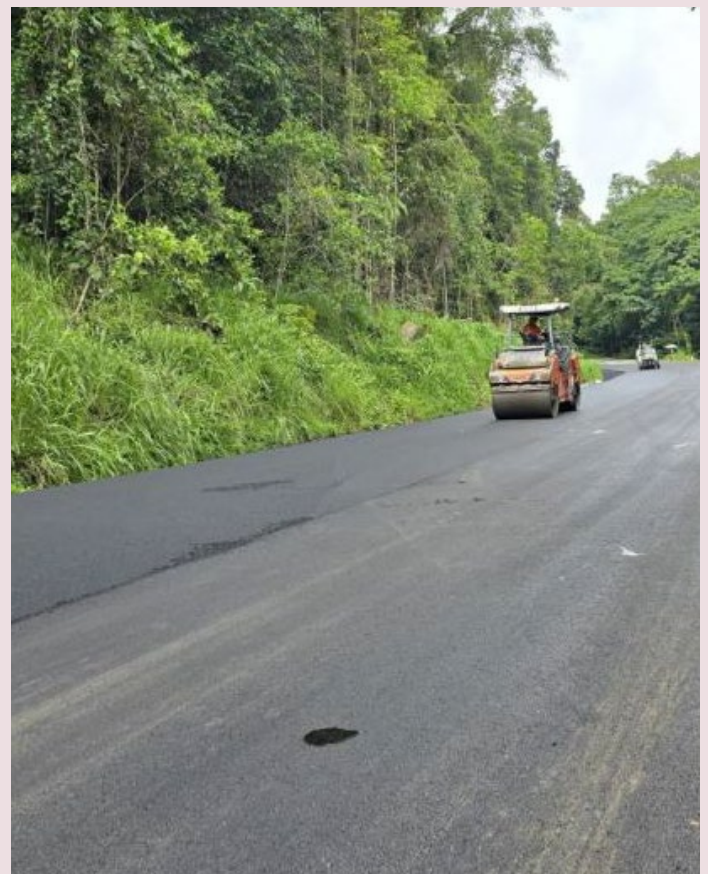
Palmerston Highway – emergency works (February 2024)
