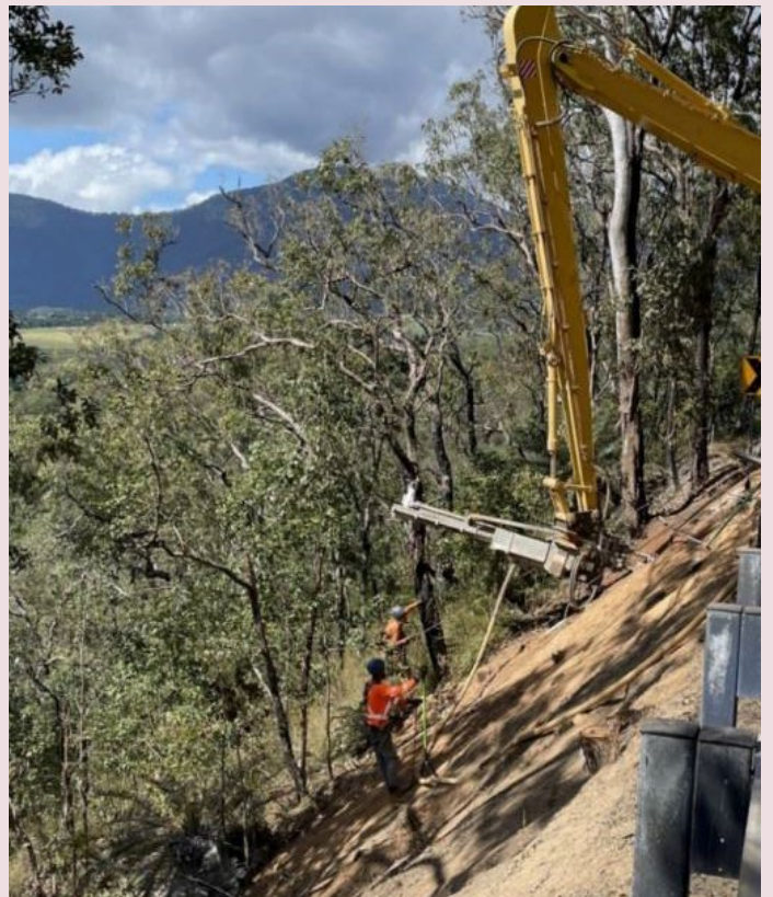
Stabilisation works in progress (July 2024)
