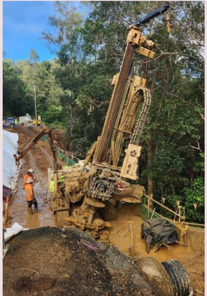
Raked pile driving in progress (May 2024)
