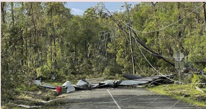
The SEQ storms caused an incredible amount of damage to the road network
