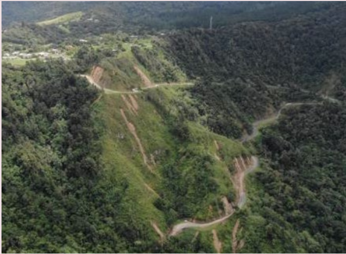
Multiple landslips caused by heavy rainfall (January 2023)
