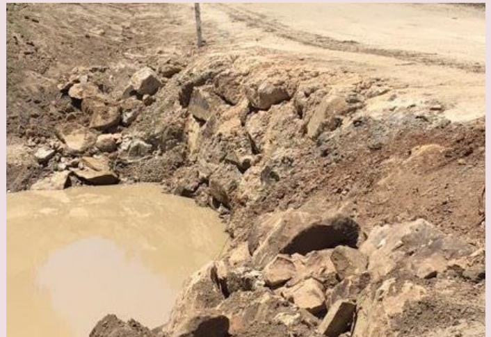
Completed emergency works at Gwambegwine Creek (Dec 2021)
