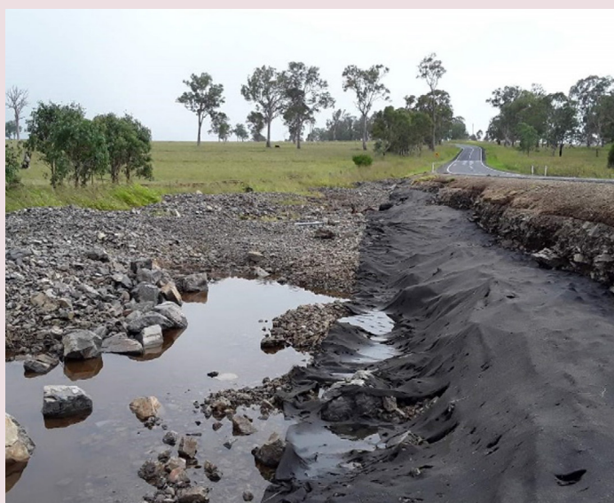
Burnett Highway (Nanango-Goomeri) – damage caused by flooding associated with Ex-Tropical Cyclone Seth (January 2022)
