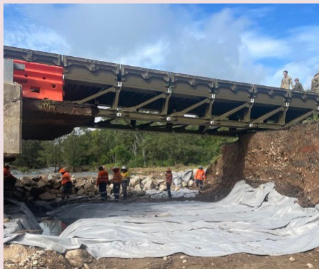
Bruce Highway (Townsville–Ingham) – temporary bridge in place at the Ed Kratzmann Bridge at Ollera Creek
