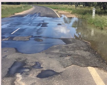
Barwon Highway (Goondiwindi–Talwood) – damage at floodway due to prolonged inundation (March 2022)
