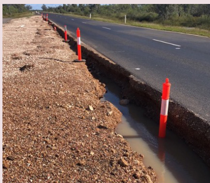
Castlereagh Highway (St George–Hebel) – shoulder scouring at floodway (May 2022)
