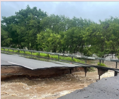
Bruce Highway (Townsville–Ingham) – severe scouring on the Ed Kratzmann Bridge at Ollera Creek
