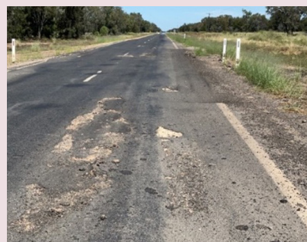
Barwon Highway (Goondiwindi–Talwood) – pavement damage (March 2022)
