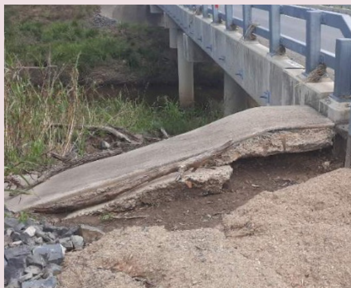
Burnett Highway (Nanango-Goomeri) – scouring at Barambah Creek Bridge caused by flooding associated with Tropical Cyclone Seth (January 2022)
