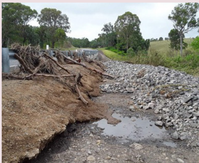
Burnett Highway (Nanango-Goomeri) – severe scouring caused by flooding associated with Ex-Tropical Cyclone Seth (January 2022)
