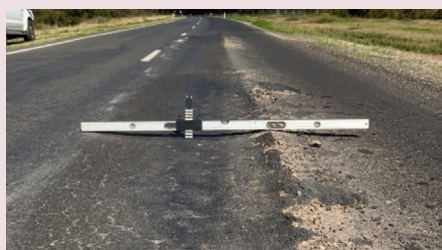
Barwon Highway (Goondiwindi–Talwood) – pavement damage from prolonged saturation (August 2022)
