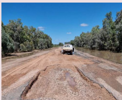
Castlereagh Highway (St George–Hebel) – pavement damage at floodway (November 2022)
