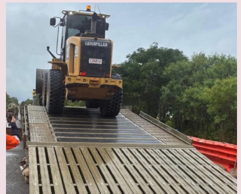
Bruce Highway (Townsville–Ingham) – temporary bridge in place at the Ed Kratzmann Bridge at Ollera Creek
