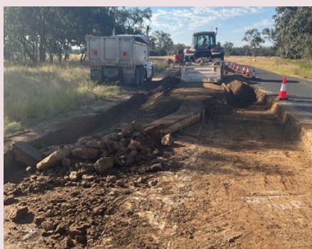
Barwon Highway (Goondiwindi–Talwood) – subgrade works at Beryl's Crossing floodway (July 2024)
