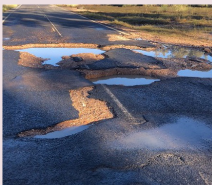
Castlereagh Highway (St George–Hebel) – pavement damage at floodway (June 2022)
