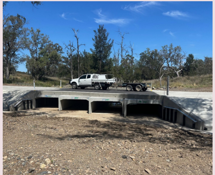
Stanthorpe-Inglewood Road – completed culvert works (January 2025)
