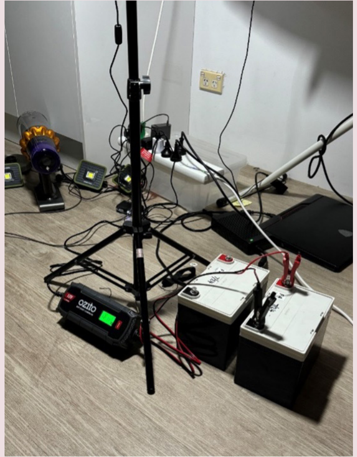
Several alternative power supplies were also organised to light common property and fire escapes, and keep the fire control panel energised
