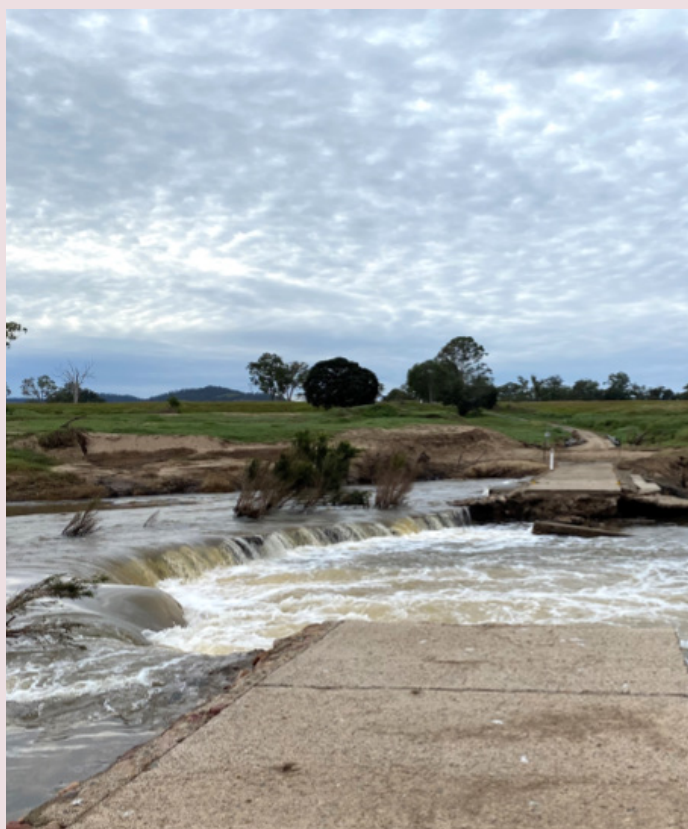
Severe flooding in February 2022 destroyed a 10-metre section of the causeway
