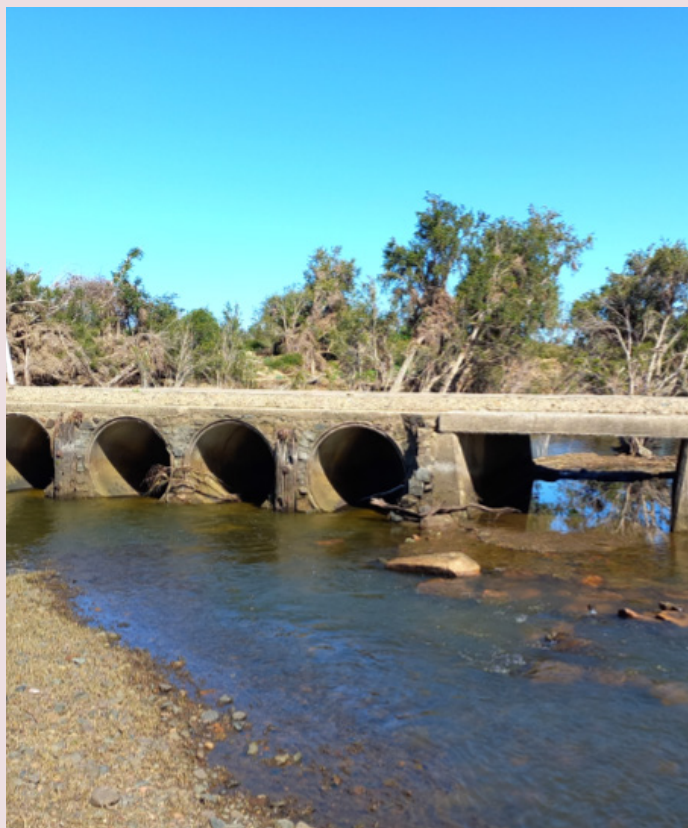
This flood-prone concrete causeway over Scrub Creek in south-east Queensland's Somerset region was regularly cut in wet weather.
