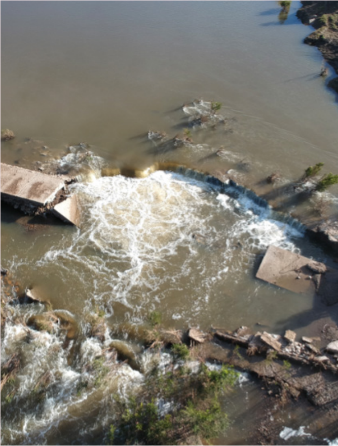
The floodwaters also washed away material beneath a section of the causeway, leaving it suspended in mid-air.
