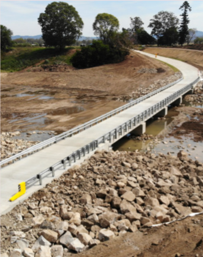
The new 30-metre-long concrete bridge has proven a game-changer for the local community and passed its first big test in December 2024, remaining open during heavy rains.
