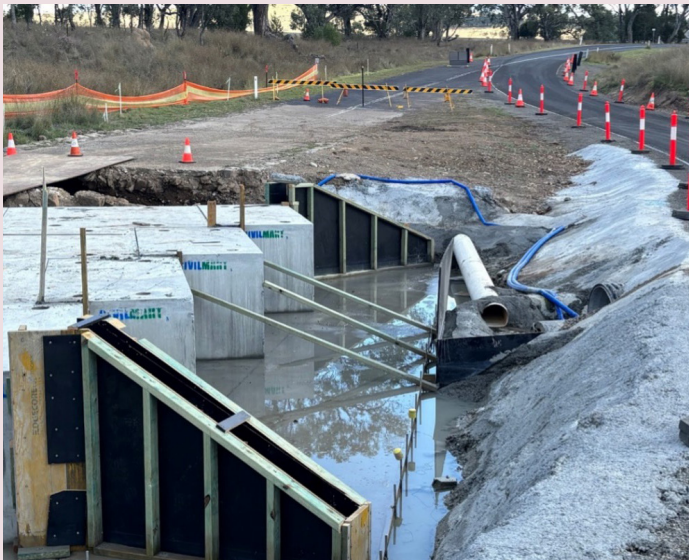
Stanthorpe-Inglewood Road – culvert works in progress, with side track and barricaded environmental area (October 2024)
