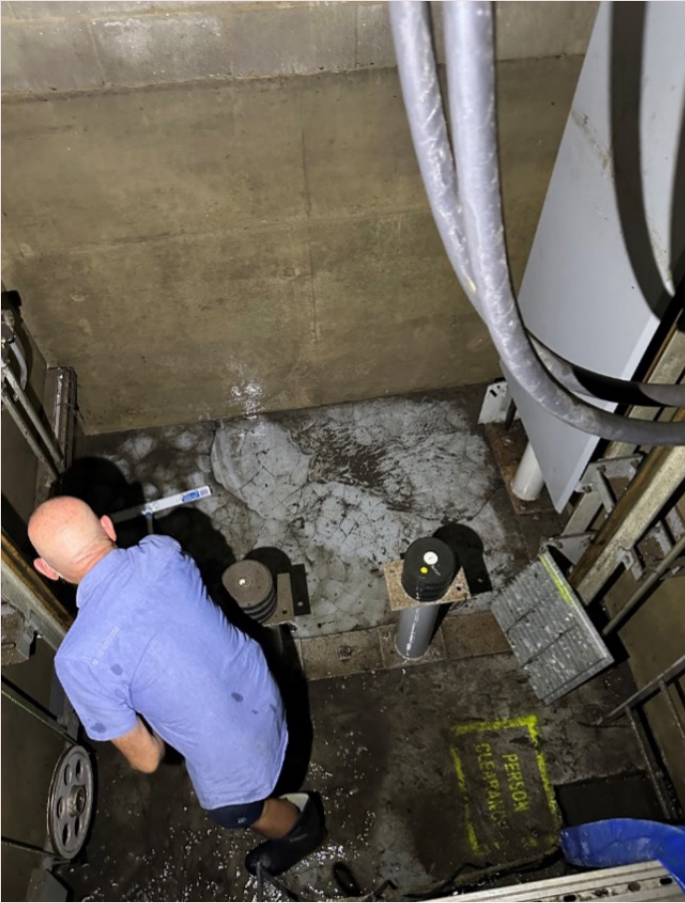
Tor hired a small pump to remove water from the resort's elevator pit then cleaned it
