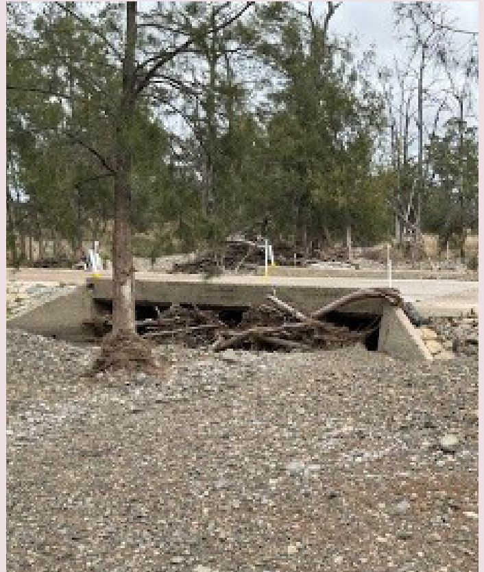
Stanthorpe–Inglewood Road – inlet damage to the culvert (October 2023)
