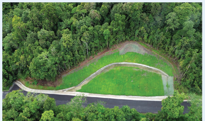
Palmerston Highway – completed works at site 2 (January 2026)
