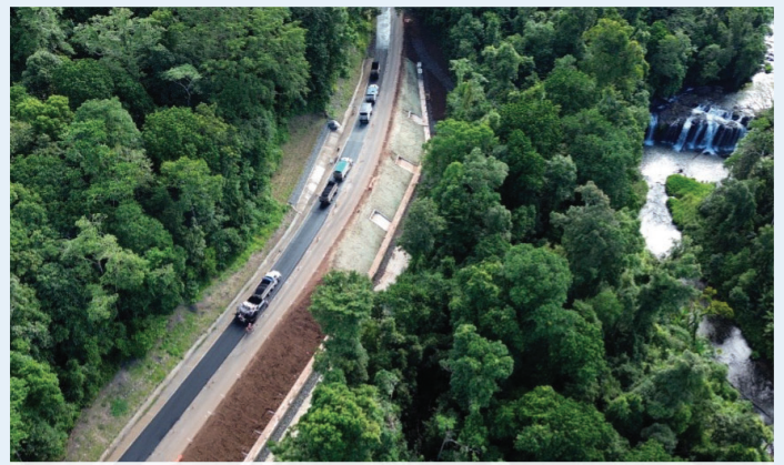
Palmerston Highway – completed works at site 1 (May 2026)
